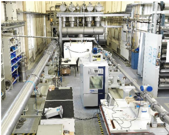
Upstream view to calibration lines
