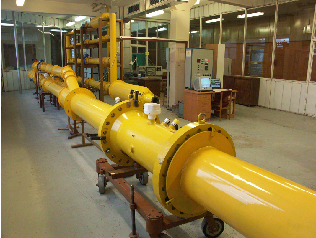
Figure 8 - The general view of the standard facility
