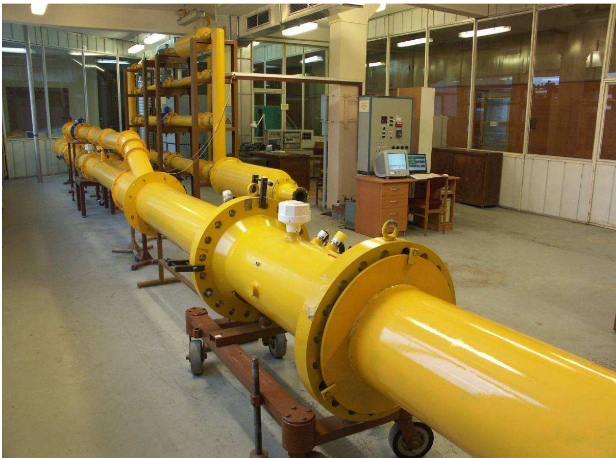
Fig.12. The general view of the standard facility
