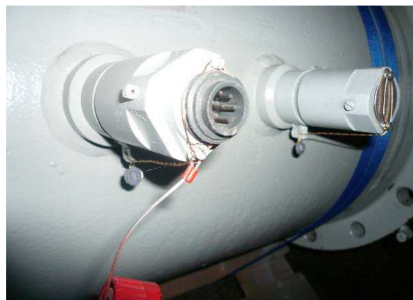
Figure 3 – Pulse emitter A1S
